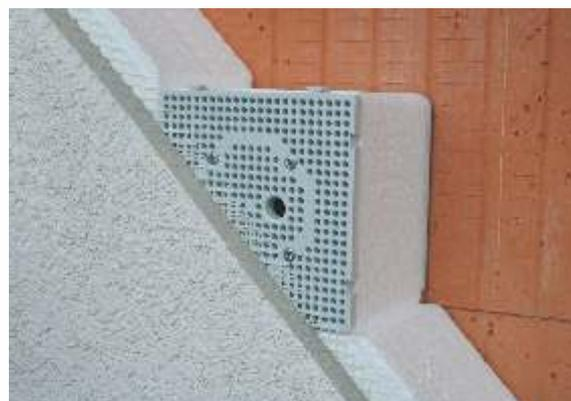
**Assembling installation box into thermal insulation MDZ 300\_KB**
