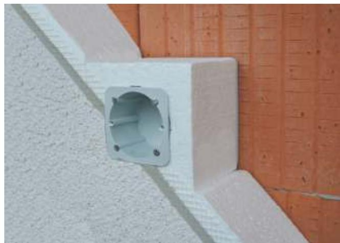
**Assembling installation box into thermal insulation KEZ\_KB**
